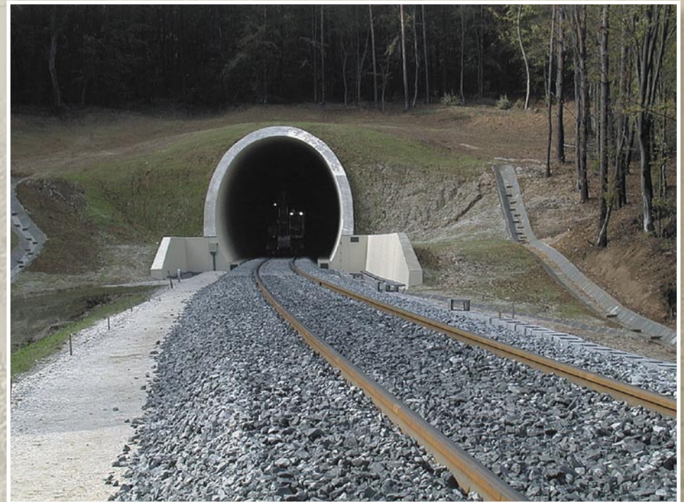
Tunel at Nagyrákos
