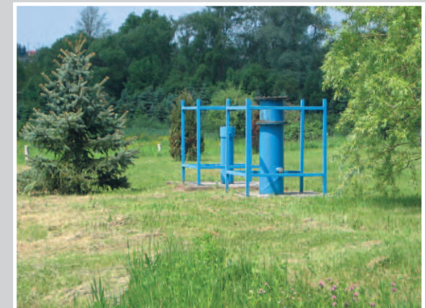
Monitoring kút Monitoring station
